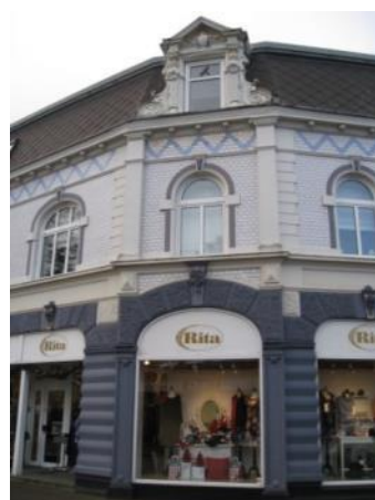
Markedsgade 32 – refendfugning, pilastre
