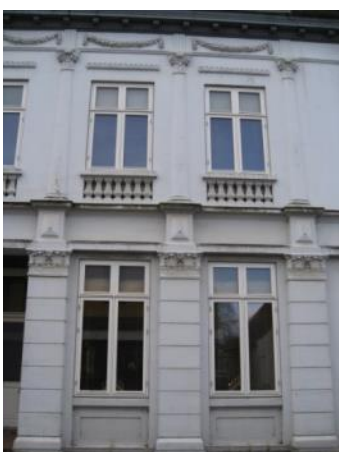
Markedsgade 28 A – kvadrefugning, pilastre, balustre under overetagens vinduer
